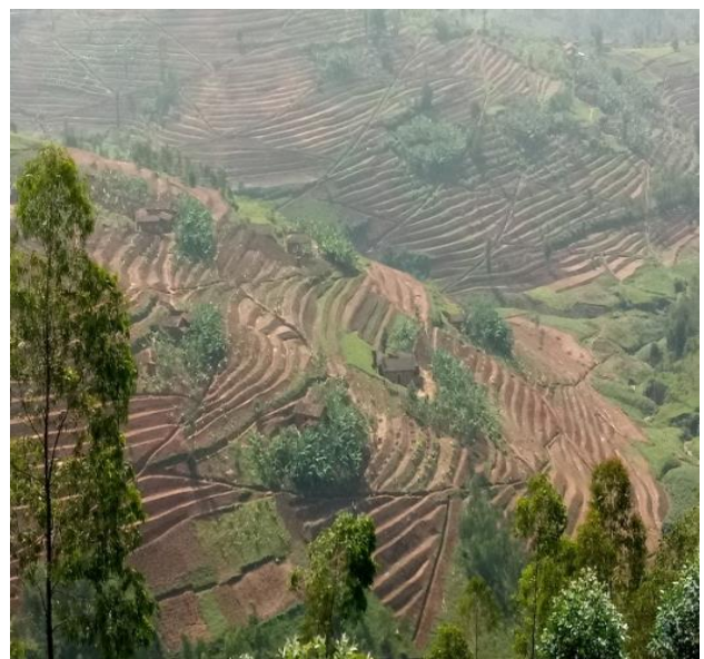
Figure 7: Picture illustrating the rehabilitation works in the Secoko Sub-Catchment with terraces.
