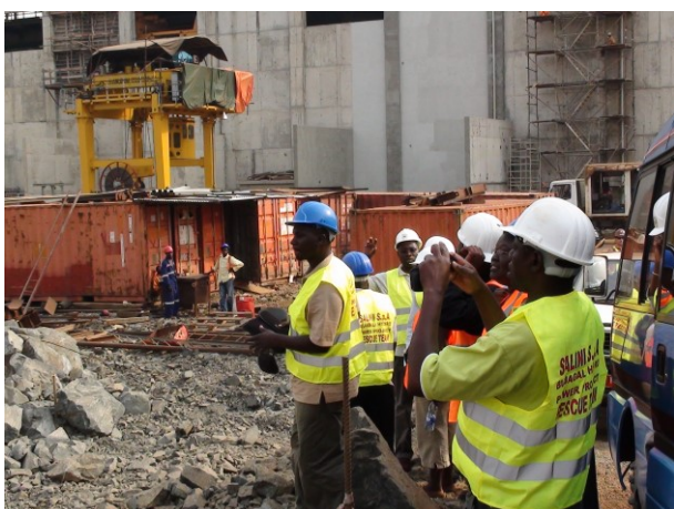
Construction of the Bujugali Hydropower dam, Uganda, 2011
