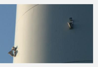
Wind turbine with a detection system at the windpark Krammer in Province Zeeland. The turbines shutdown whenever a bird, such as the protected white-tailed eagle, is within 600m range from a turbine.
